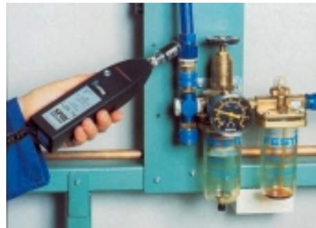
Leaks in pressure and vacuum systems
